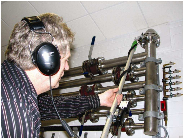
Picture 10 Checking for leakages in flanges
