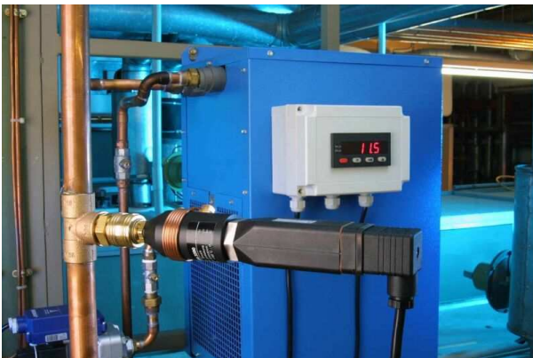
Picture 11 Continuous dew point control
