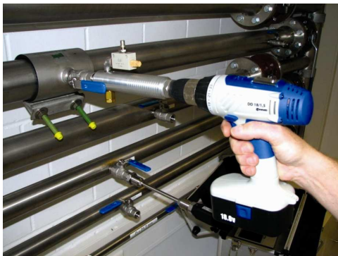
Picture 6 Drilling under pressure
