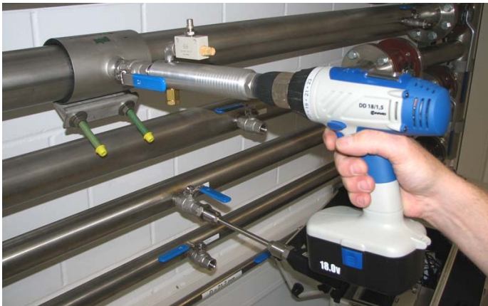
Drilling with CS drilling jig Order no. 0530 1108
