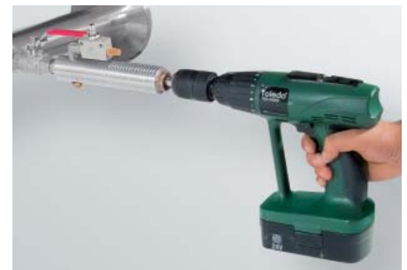
Drilling under pressure
