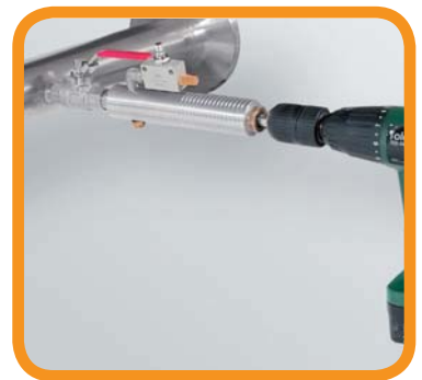
Drilling under pressure
