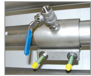
B Spot drilling collars
