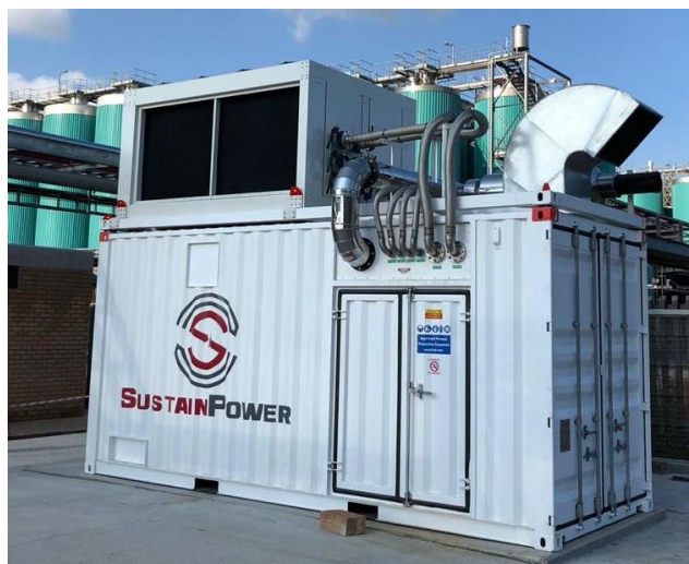
Figure 3: Containerised CHP unit at Distell Springs © CS SustainPower
